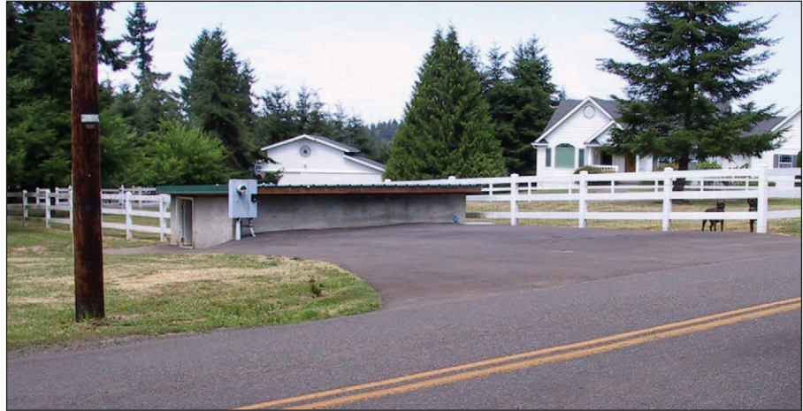
The ASR well for McNulty Water People's Utility District in Warren, Oregon, holds 6 million gallons of water, six times the storage capacity of its three above-ground reservoirs, and does so without significantly impacting the scenery in the area. Photo by John Borden.
